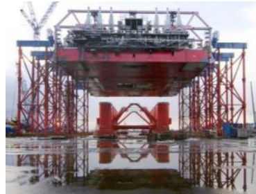
SARENS MULTI LIFTING TOWER
