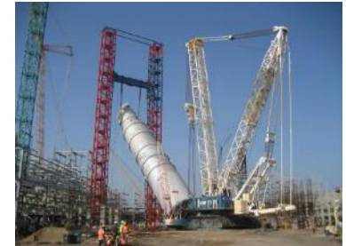
SARENS CLIMBING TOWERS
